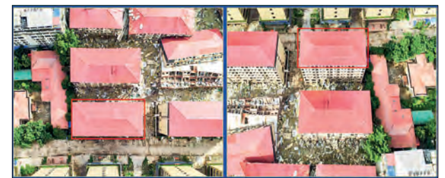
Images show the update before and after the demolition of the seven-storey scam hub.
