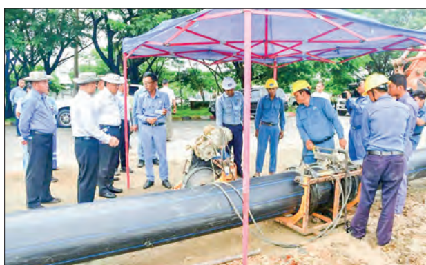
This photo features a new HDPE pipeline to be installed to replace the water supply system from the Chaungmagyi Dam.
